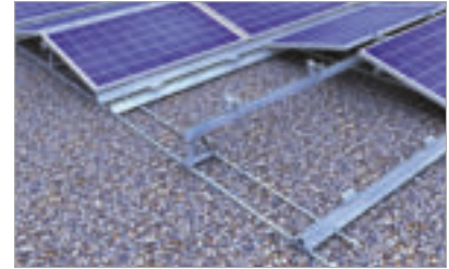
Flat roof I
